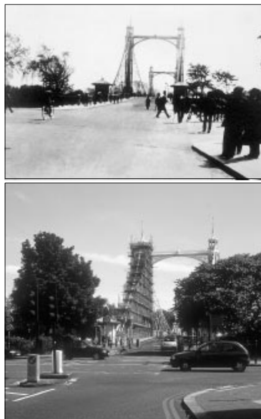
Fig 4 Albert Bridge, Chelsea c1900 (top) and 2000 (bottom). The main change is that the trees have grown: 100 years is long in the lifespan of humans but not in that of a city
